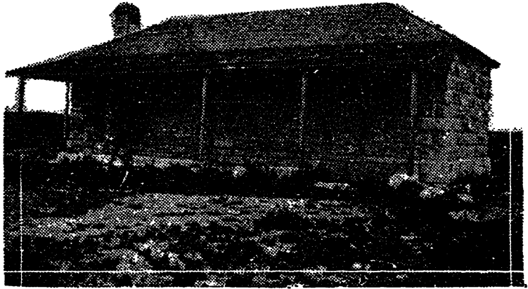
FORT STOCKTON GUARD HOUSE
