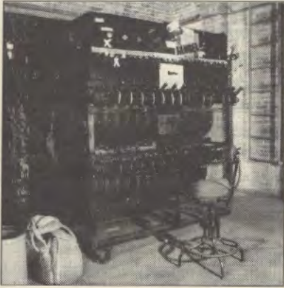
Original remote controlled stage lighting console, which remains intact to this day. El Paso Public Library Archives
