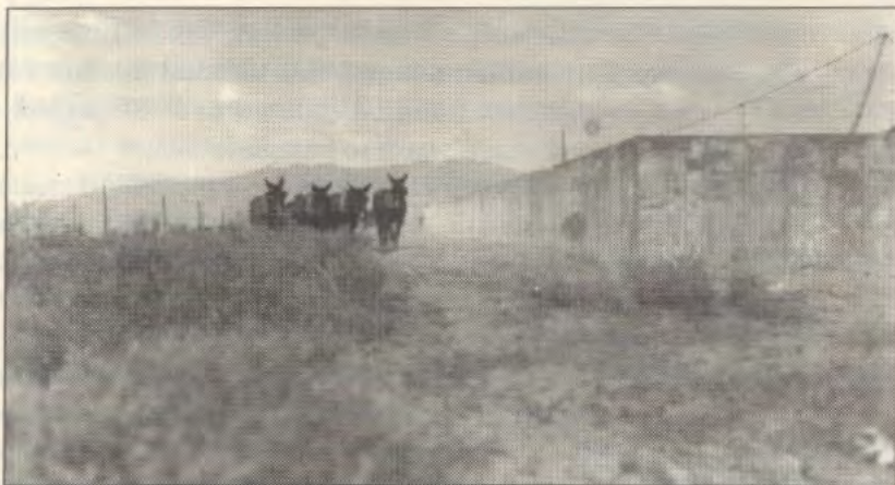
Mules belonging to Chris P. Fox doing excavation work.
