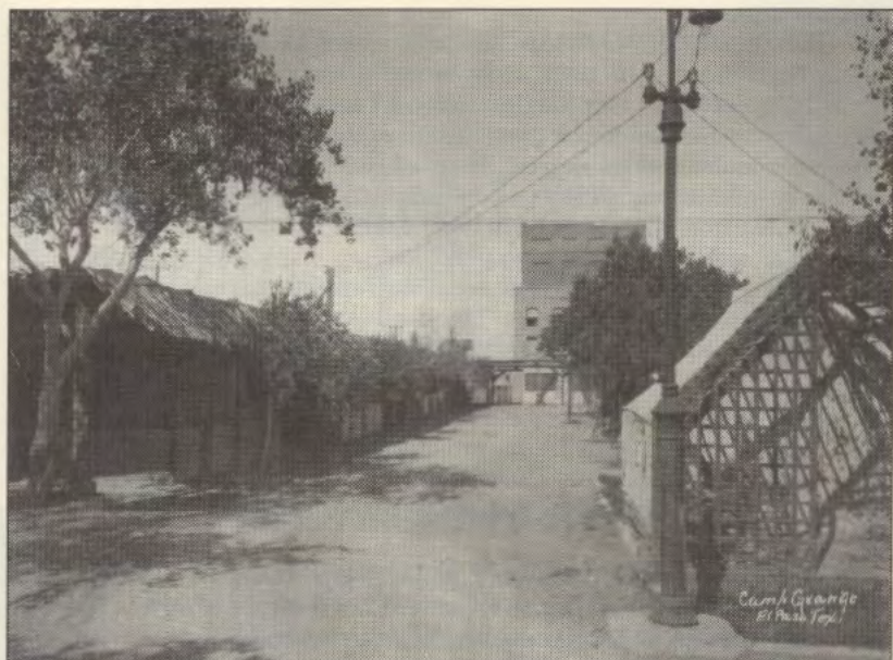
The old Harry Mitchell's Brewery looms upward at the north end of the road that wound through Camp Grande.
