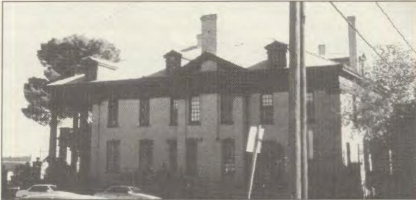
1011 North Mesa · The north and west walls which show the size of the house (Dec. 2000)
