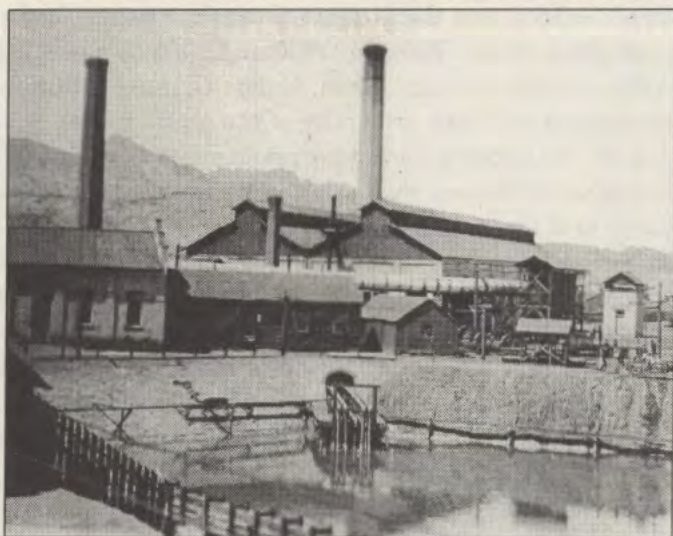
Several ponds were on the ASARCO property. All but one were used for drainage for the various processes. Note in the center the drainage pipe coming from the building into the pond.
