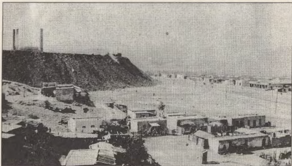
Houses were very near a slag heap.
