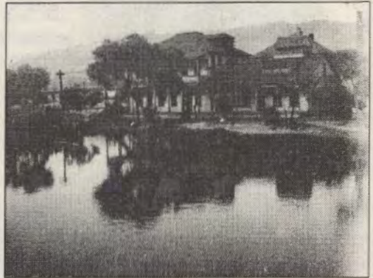
The smelter offices were next to one of the ponds.
