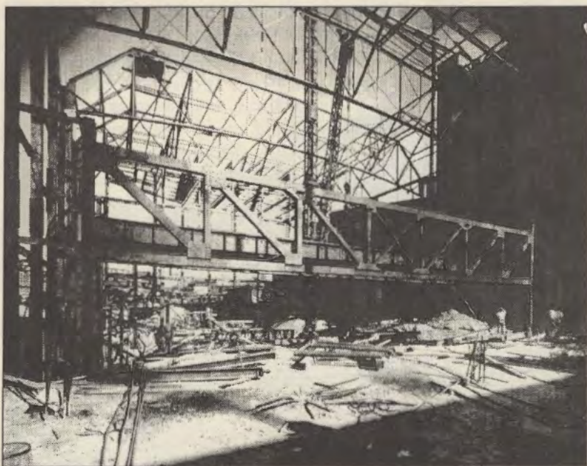
The largest I-Beam in Texas supports the balcony.
