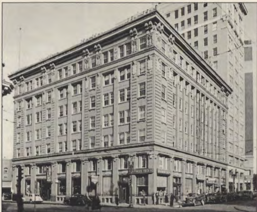
The American Furniture Company Building on the northwest corner of Oregon and San Antonio Streets before its façade was modified. The Texas Tower can be seen in the background. Courtesy of the University of Texas at El Paso Library, Special Collections Department, J.E. Morgan & Sons photographs, PH020.
