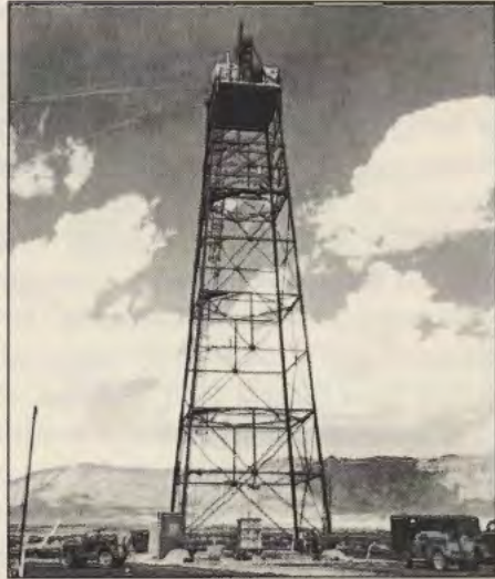
The tower used to test the first atomic bomb at the Trinity Test Site in New Mexico. Courtesy of the University of Texas at El Paso Library, Special Collections Department, J.E. Morgan & Sons photographs, PH020.
