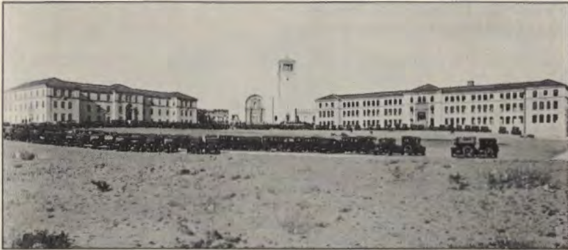
Loretto Academy circa 1924. Most of the original buildings have been completed, but there is still some construction taking place to the left of the chapel. Courtesy of the University of Texas at El Paso Library, Special Collections Department, J.E. Morgan & Sons photographs, PH020.
