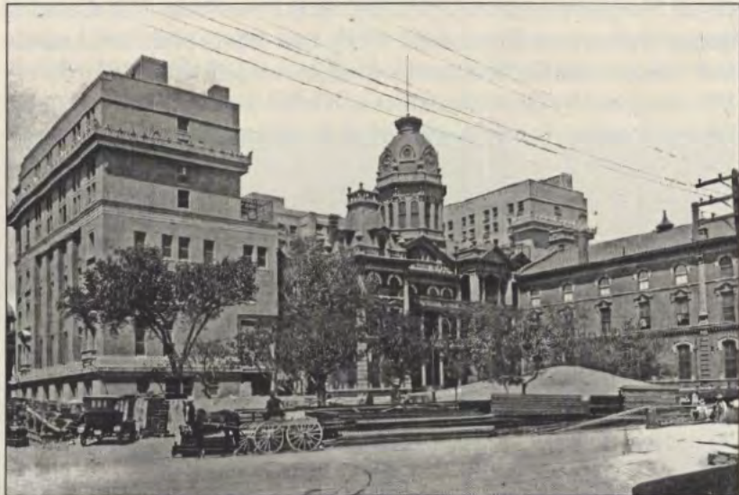
The back side of the newly completed El Paso County Courthouse, 1917. As can be seen in this photo, J.E. Morgan built a new courthouse around the original one, which had been constructed in 1885. Morgan then razed the old courthouse and replaced it with Liberty Hall. Courtesy of the University of Texas at El Paso Library, Special Collections Department, J.E. Morgan & Sons photographs, PH020.
