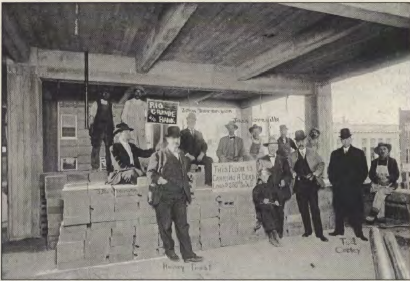
The Abdou Building under construction in 1909-1910. Joseph Morgan is left center, sitting cross-legged on a stack of bricks, holding a sign that reads "Rio Grande Valley Bank and Trust" (the original name of the building). Henry Trost is standing in the foreground to the right of Morgan, with his right hand in his pocket. John Sorenson is sitting in the background to the right of Morgan and Trost, his head slightly to the right of the sign. They were on the second or third floor of the building and the photographer was looking northeast; the white building in the background on the right is the R.B. Stevens Building, located on the corner of Mesa Ave. and Texas St. The sign on the bricks reads "This floor is carrying a dead load of 250 lbs. per square foot." The Morgan firm often tested materials as it built, especially when constructing innovative designs with new materials. Courtesy of the University of Texas at El Paso Library, Special Collections Department, J.E. Morgan & Sons photographs, PH020.
