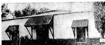
AGE A MYSTERY—The Valley Inn, Ysleta landmark, doesn't look its age which is well over 100 years but how many more, on one answer exactly. The exterior is white stucco with brick around the lower part of the building. Windows are on the overhang above the windows and front door. The roof is made in the Spanish colonial style with cast-iron beams, white stucco and a red tile roof with a fast thickness of dirt.
